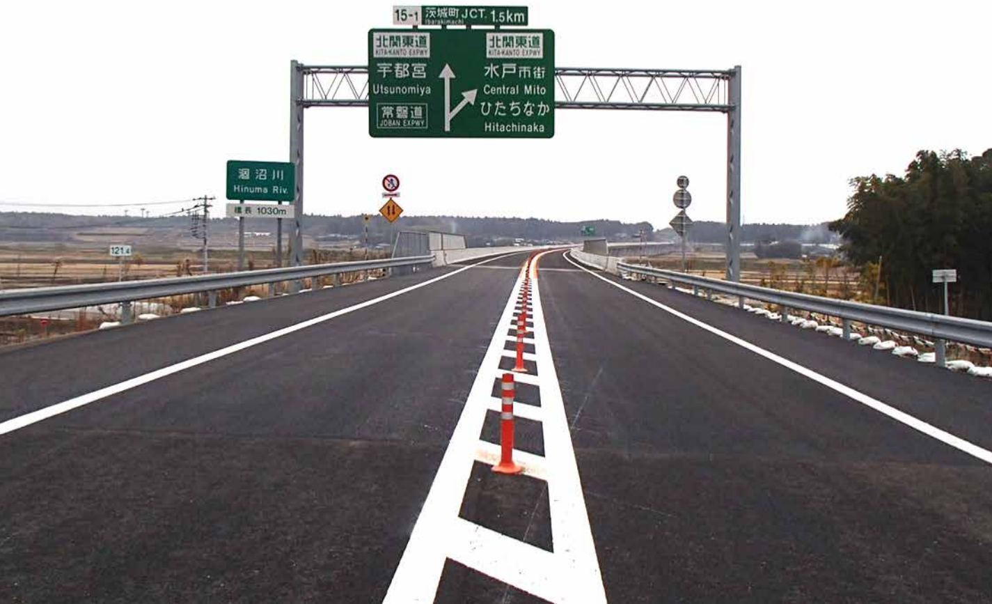
MITO, KITA KANTO EXPRESSWAY
